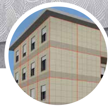
The red lines indicate the correct position of the elastic divider joints on façade coverings.
